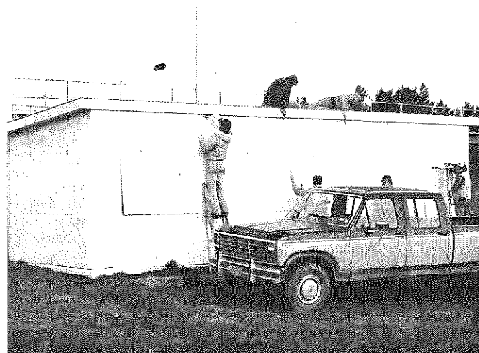
Track Construction - Workers perform maintenance on the concession stand behind the pits, in preparation for the coming season. Ade Ketchum Photo
